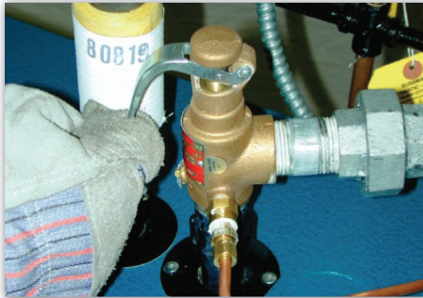
Testing a Steam Release Valve
